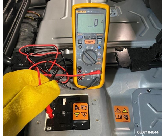
Figure 9 – HV Battery Test Points
