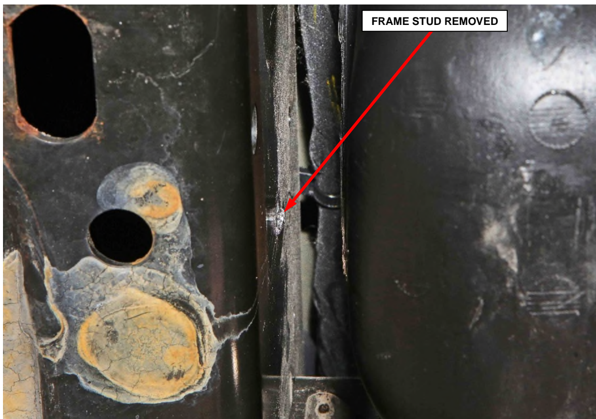
Figure 8 – Frame Stud Removed
