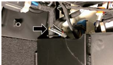
Auxiliary Switch Connections – Passenger Side Panel
